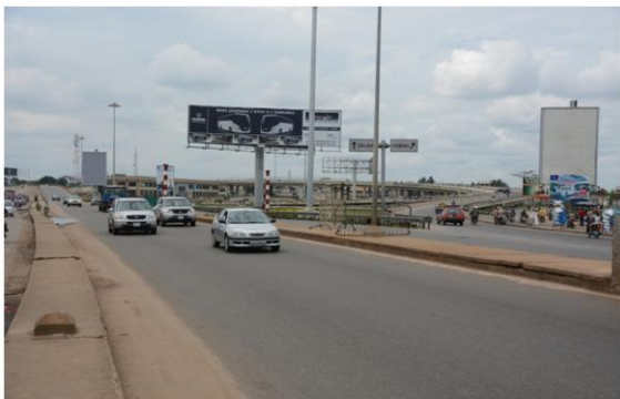
Figure 7: New Godomey Interchange (Photo: D. D. BOKO-HAYA)
